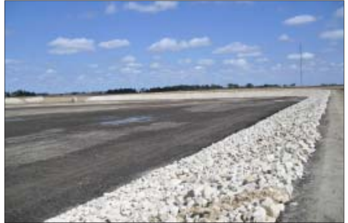
Construction on Newell wastewater project nears completion.
